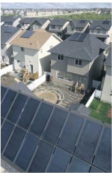
The heating for 52 homes of Drake Landing almost exclusively comes from solar energy. SUPPLIED
