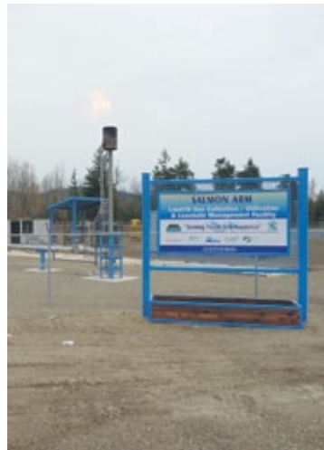
The Salmon Arm landfill gas collection facility. SUPPLIED
